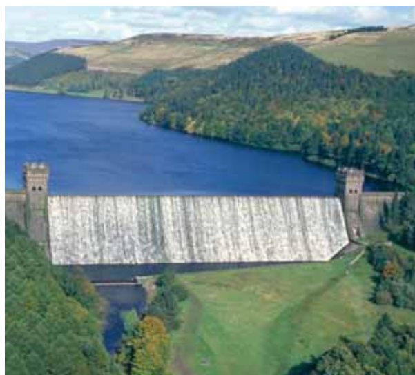
Severn Trent Water Authority
